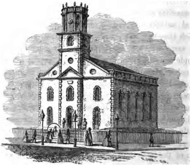
St. George's Chapel in Beekman street, erected in 1752.
